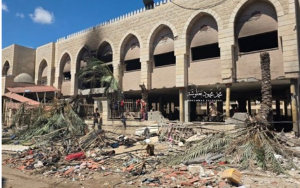
Israel eliminated 31 terrorists meeting in a room in the corner of this Gaza school building—see blackened section, upper left. Hamas originally claimed more than 100 were killed—a fact Western media reported without confirming. Why were terrorists meeting in a school?
